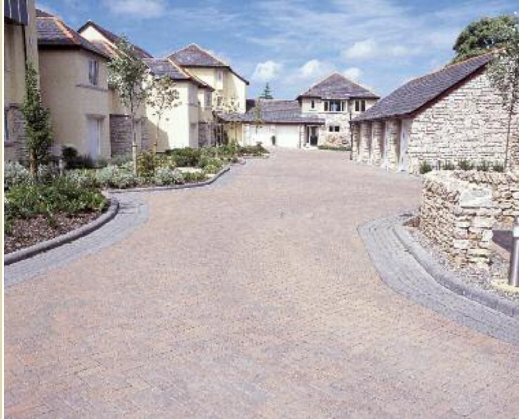
Left: Lakeland Driveway in Brindle with Charcoal border and edged with Lakeland Q Kerb in Charcoal Below: Lakeland Driveway in Buff Right: Lakeland Driveway in Red
